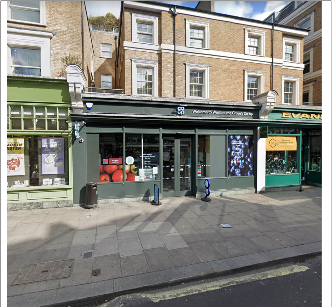
Front of Application Site
